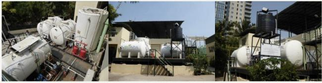
Figures 5, 6 and 7: Combined wastewater treatment system (SBR and MBR) for wastewater reuse in Amanora Park Town (source: BIOAZUL, 2015)
